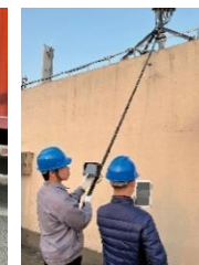
constructure inspection (WIFI real-time image transmission)
